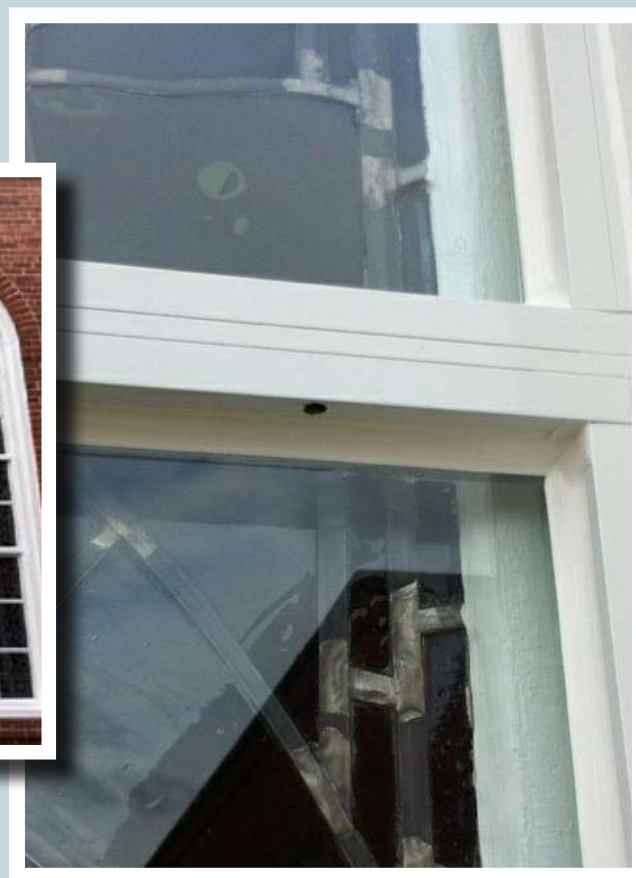
Right: A discreet venting system was used in the frame work to allow heat to escape
